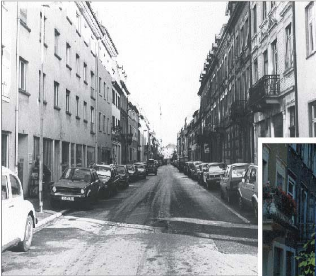
Typical residential street in Freiburg BEFORE traffic calming reforms
