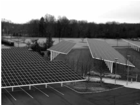
Installation of solar carports.
