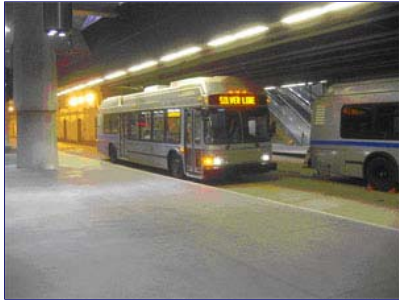
The Silver Line's exclusive right-of-way tunnel.
