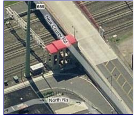
Stairway provide pedestrian access to Secaucus Junction (connecting New County Rd with North Rd)
