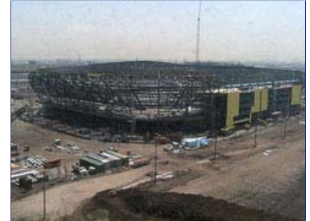
Under Construction Red Bull Arena
