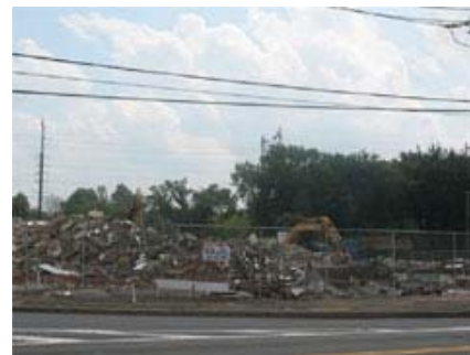
Demolition and clearance, July 2009
