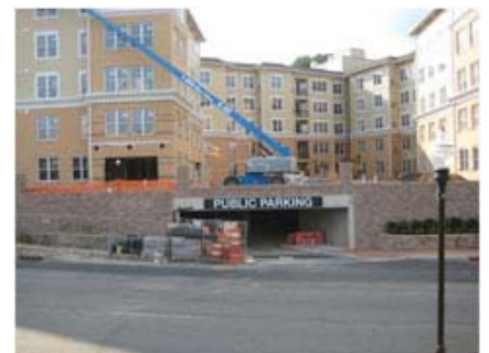
Construction Over and Around the Recently Completed Morristown Parking Deck
